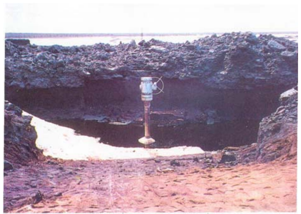
FIG. (22-H) THE WELL HAS BEEN SUCCESSFULLY CAPPED
