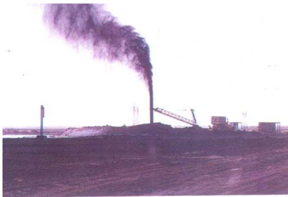
FIG. (22-G) THE FIRE HAS BEEN SUCCESSFULLY EXTINGUISHED AND THE WELL HEAD IS PREPARED FOR CAPPING.
