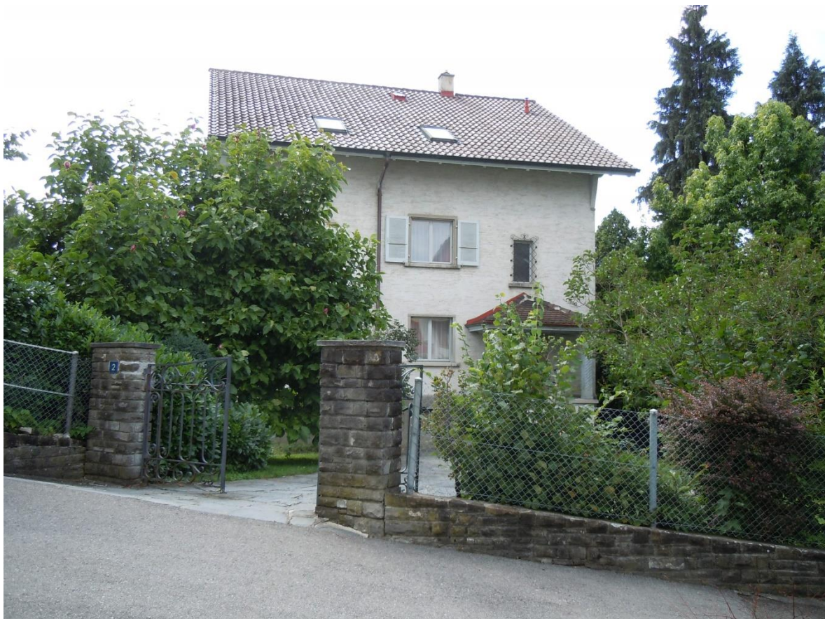
Access to the villa from the east
